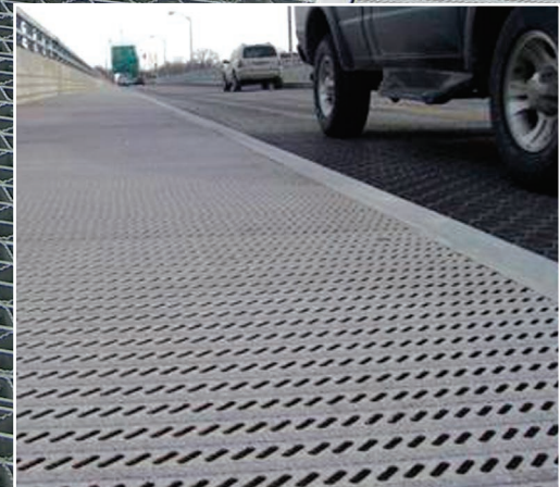
Grosse Ile Bridge, MI - Aluminum Plank Walkway
