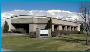
INTERSTATE GRATINGS, UT ▲
